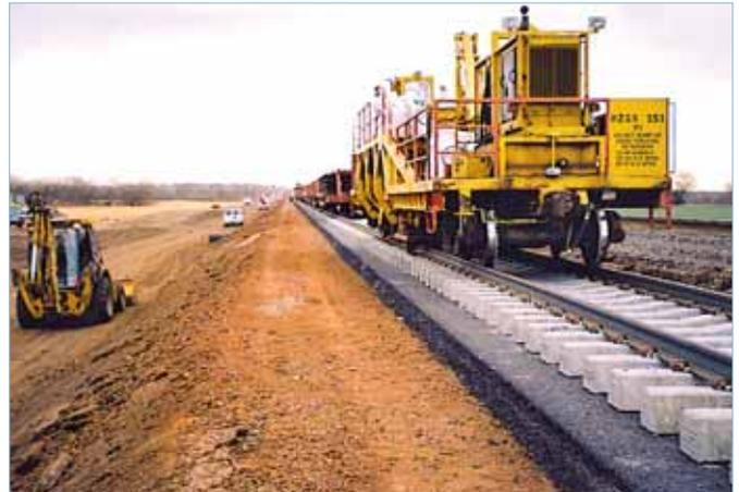
Positioning a new track on the BNSF transcon project prior to adding the ballast and 'pulling the track up' to achieve the desired thickness of ballast.
