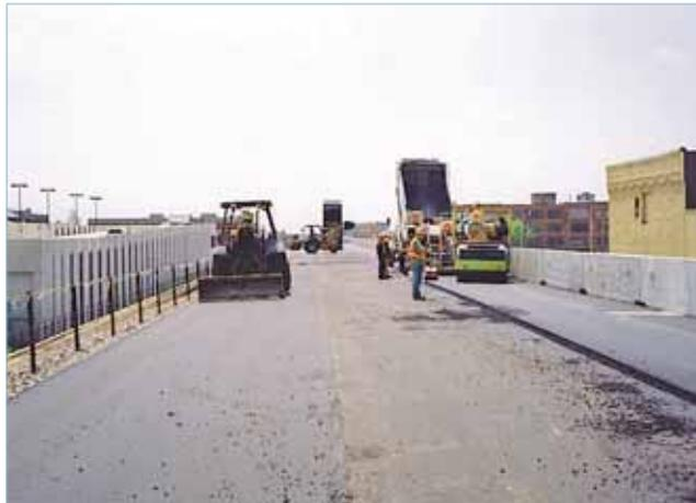
Placing asphalt underlayment on the Wichita, KS elevated track section for the mainlines of the BNSF and UP railways.
