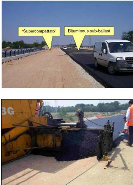
**Figure 5. Installation of asphalt trackbed layer.**
