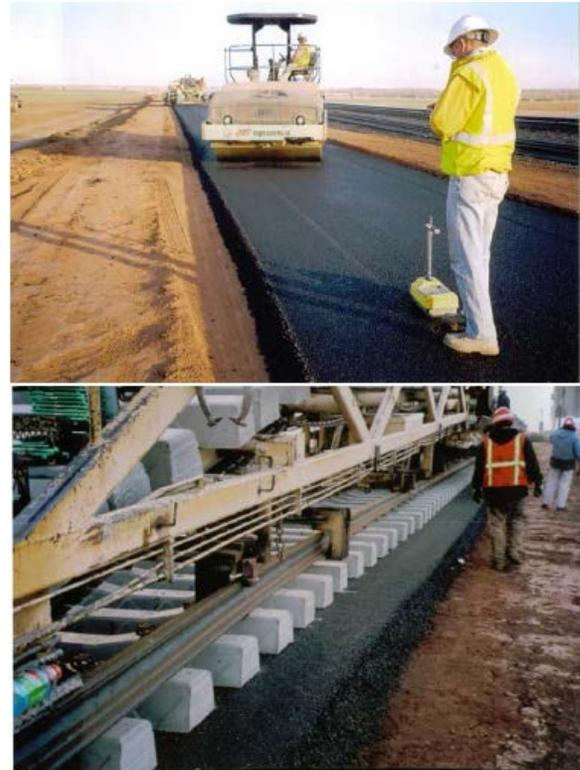
**Figure 1. BNSF Transcon asphalt trackbed construction.**
