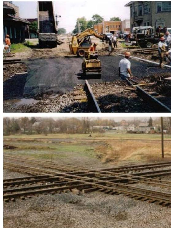
Figure 6. CSX 4-diamond rail crossing installation in Chicago.
