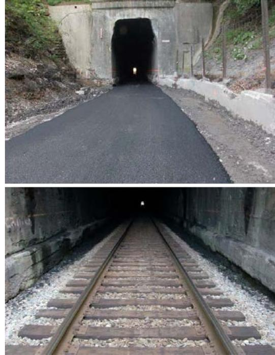
**Figure 3. NS Heartland Corridor tunnel floor construction.**
