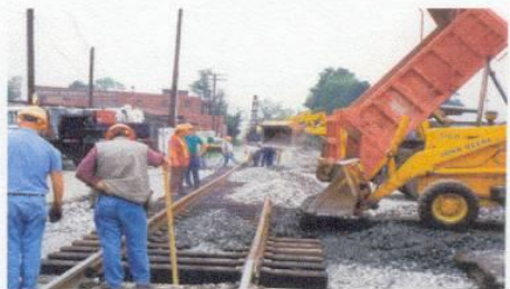
Dumping cribbing rock
