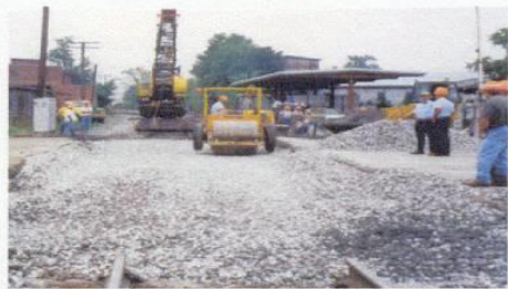
Compacting ballast
