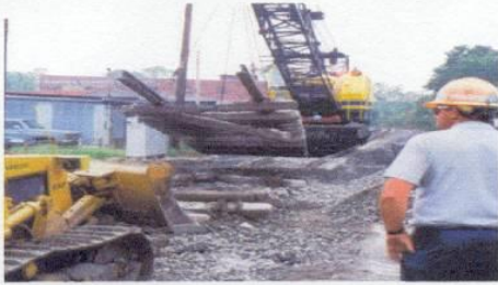
Lifting out old Panel
