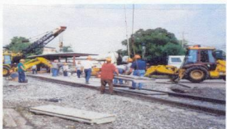
Placing concrete surface
