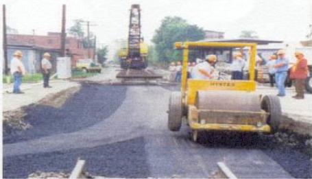
Compacting asphalt
