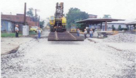
Positioning wood tie panel
