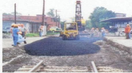
Compacting placement of asphalt
