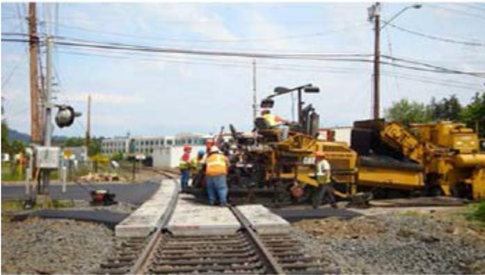
**Figure 9. WES Commuter Line Crossing (SW Durham Road) on Portland & Western RR near Portland, OR, one of 13 Crossings Underlain with Asphalt.**
