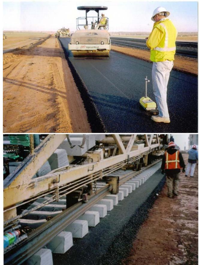
Fig. 4. BNSF Transcon asphalt trackbed construction. UP/BNSF Grade Separation Project
