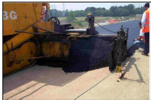
Fig. 3. Italian asphalt trackbed construction.
