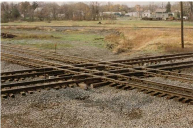
**Fig. 9. CSX 4-diamond rail crossing installation in Chicago.**
