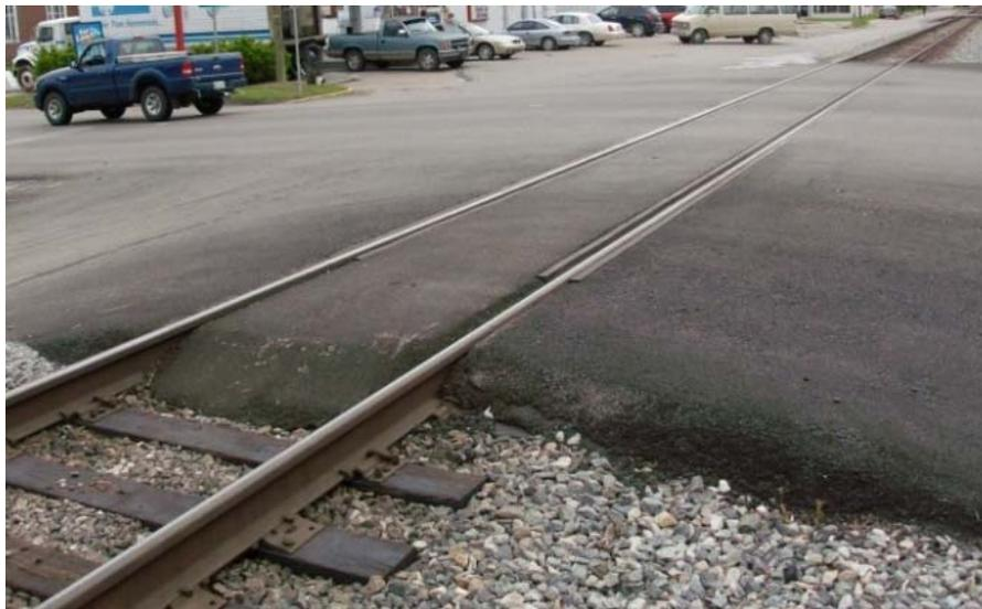
**Typical Rubber/Asphalt Crossing Surface**
