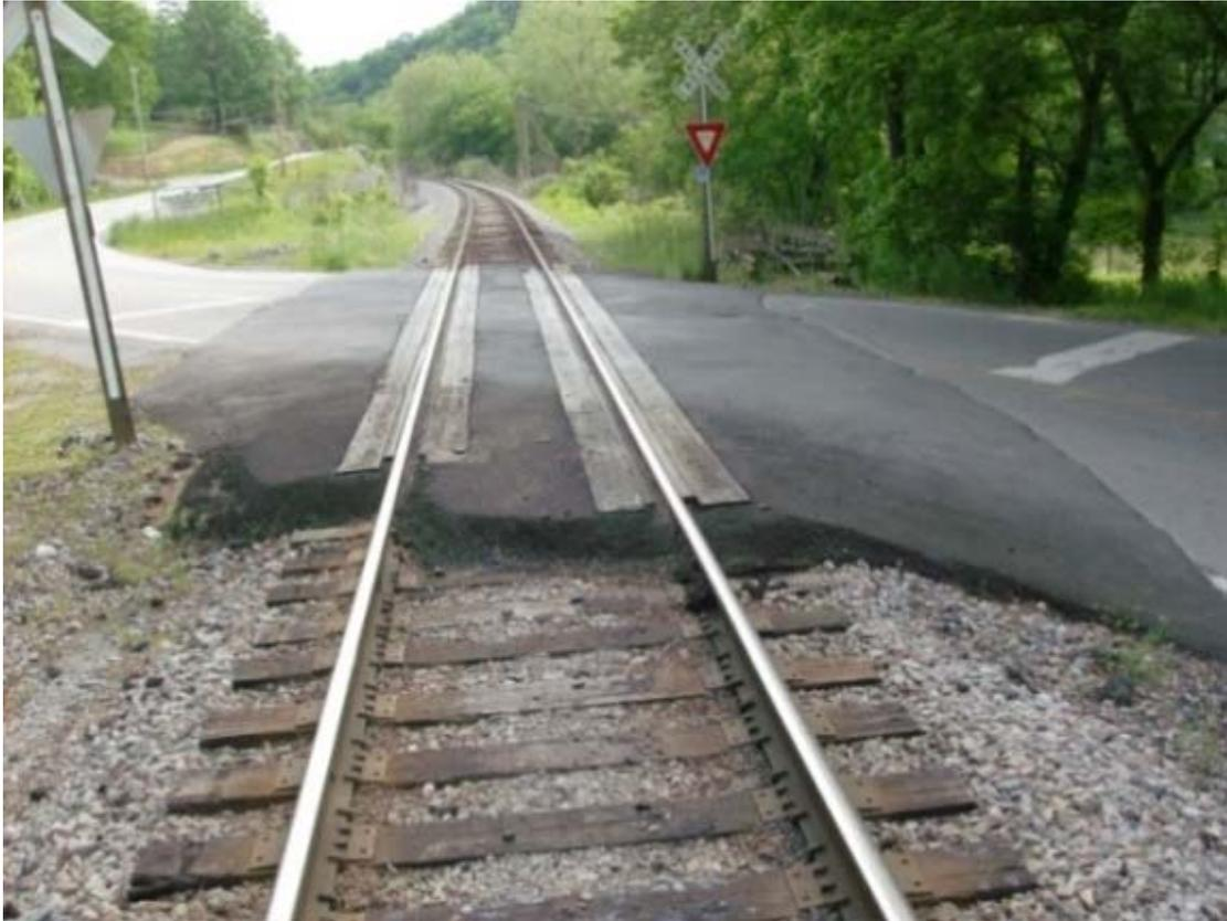
**Typical Timber/Asphalt Crossing Surface**
