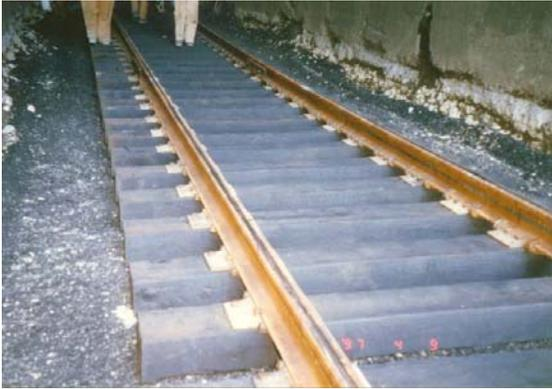
Figure 4. New track panel on compacted HMA tunnel floor prior to adding ballast and raising track
