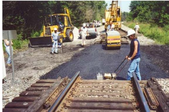
Figure 8. Compacting HMA underlayment bridge approach approach prior to adding ballast and track panel
