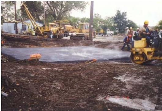
Figure 10. HMA underlayment for 4-diamond renewal prior to adding ballast and trackwork
