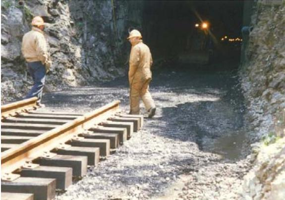
Figure 3. Placing HMA in tunnel portal
